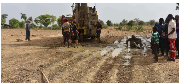
On-going Water Point drilling in Zuru LGA, Kebbi State.
